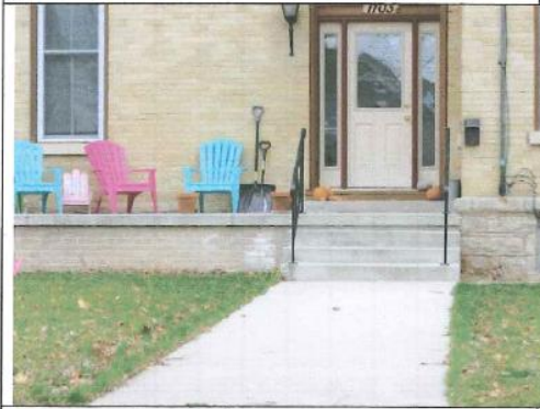
Fig.3 Nearby terrace/ Chapin Street
