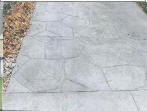
Fig.4 stamped concrete – sample of contractors work Nelson GC
