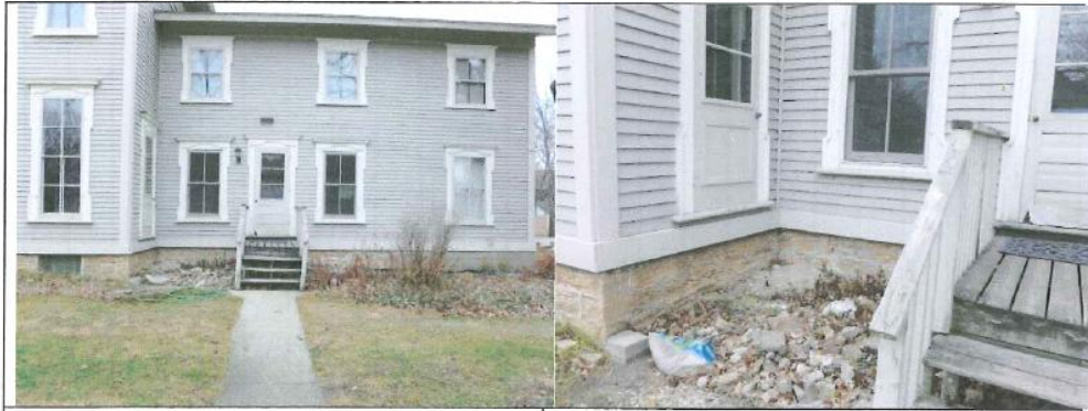
Fig. 1: Current stairway, Chapin Street entrance.
