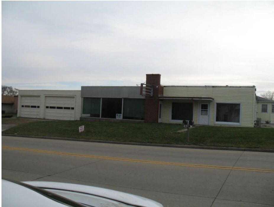
Figure 1: North view of property from Liberty Avenue
