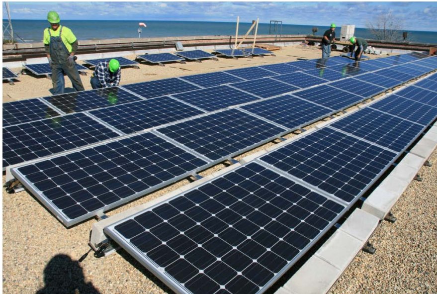
Figure 6 Solar Panel Array Assembly
