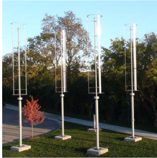
Figure 2 Vertical Axis Turbines at Devon Bank of Wheeling, Illinois (Windspire Energy)
