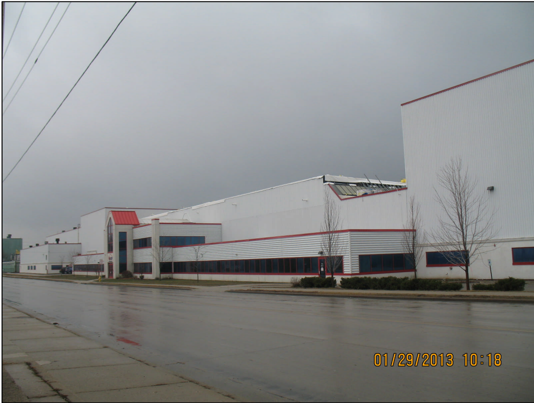
ACM Property Located West of Grocery Store
