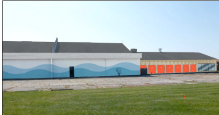
VIEW SIDE- BLDG. 'A'
