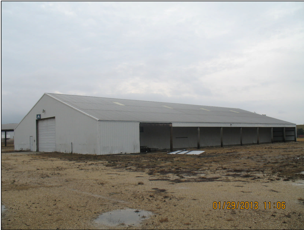
Detached Accessory Structure a/k/a Building “C”
