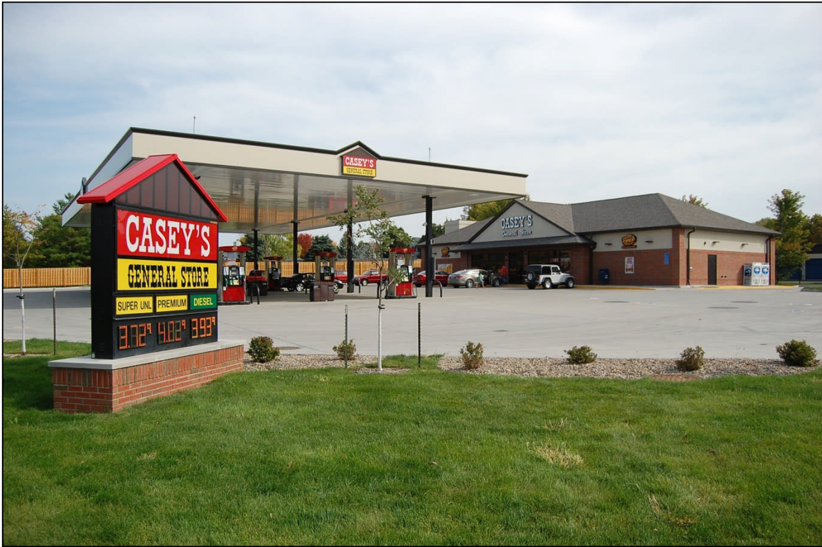
Casey's General Store with Gas Island Canopy and Primary Ground Sign
