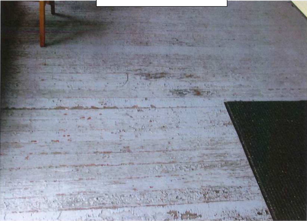
717 Emerson Street, Porch Repairs
