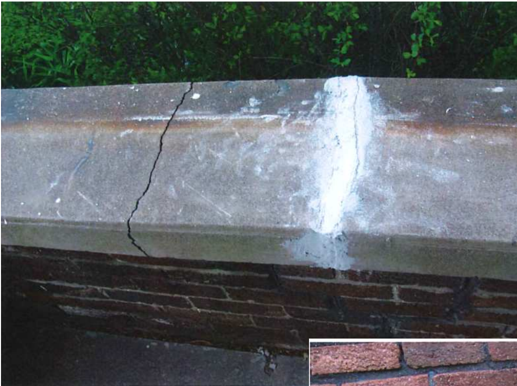
619 College Street, Porch Repairs
