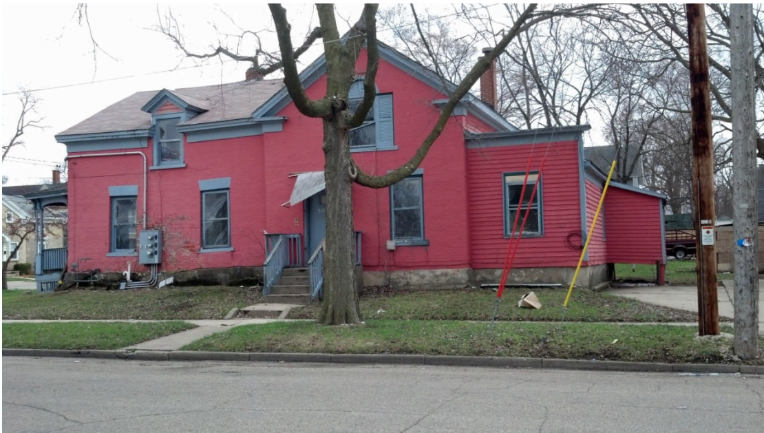
422 Bluff Street - North Side
