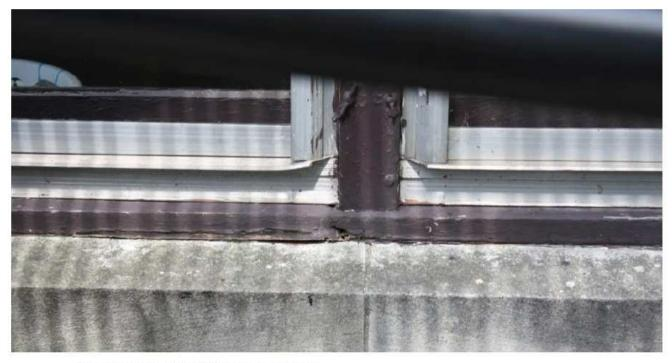
South side 1st floor behind fire escape, sill damage
