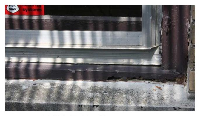
South side 1st floor further sill damage detail
