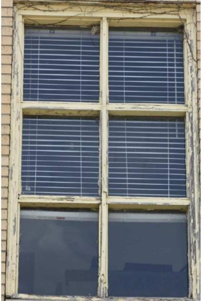
East side 1st floor window showing dry rot
