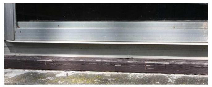
South side 1st floor next to back door, sill damage
