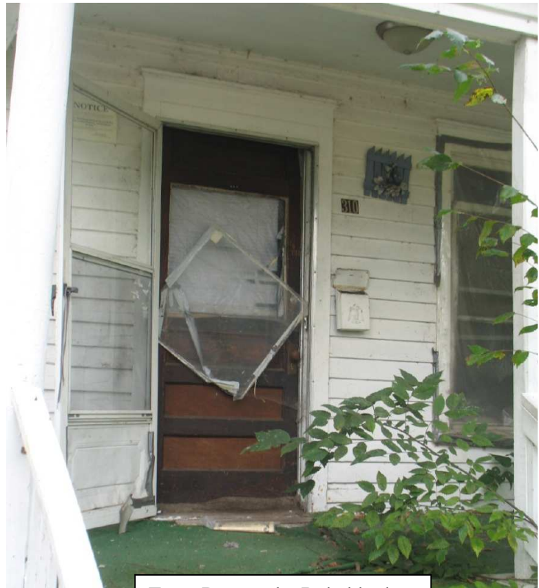
Front Door to be Rehabbed
