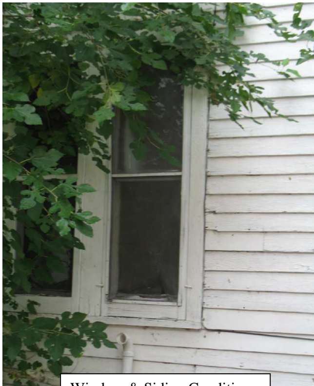
Window & Siding Condition
