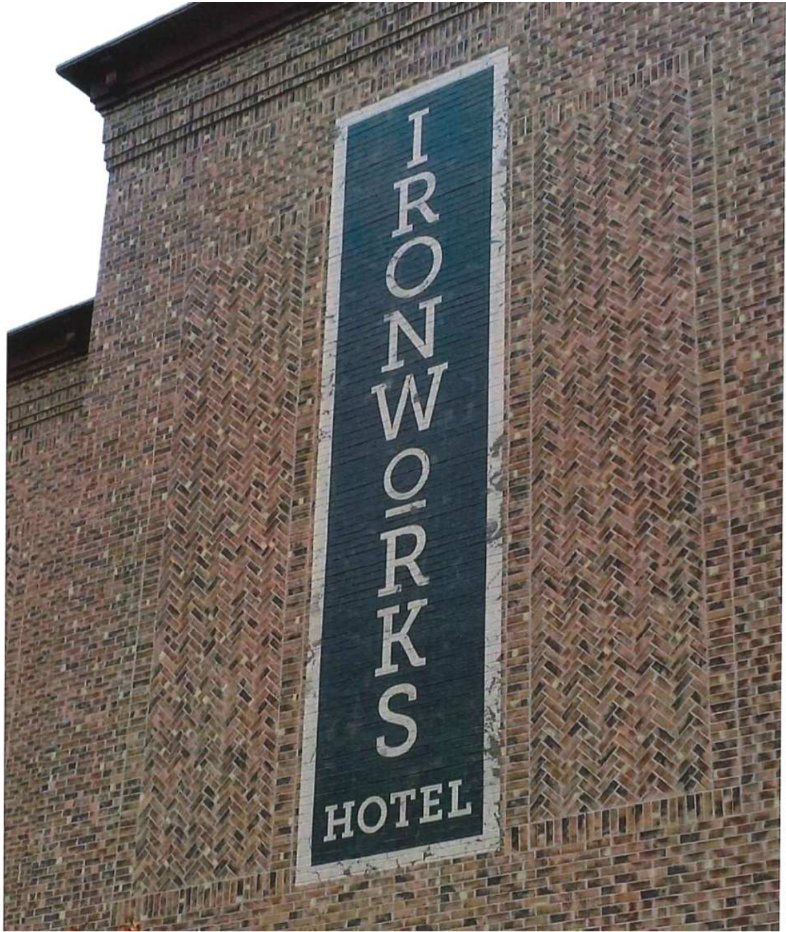
Vinyl wall signs installed on the North and South elevations
