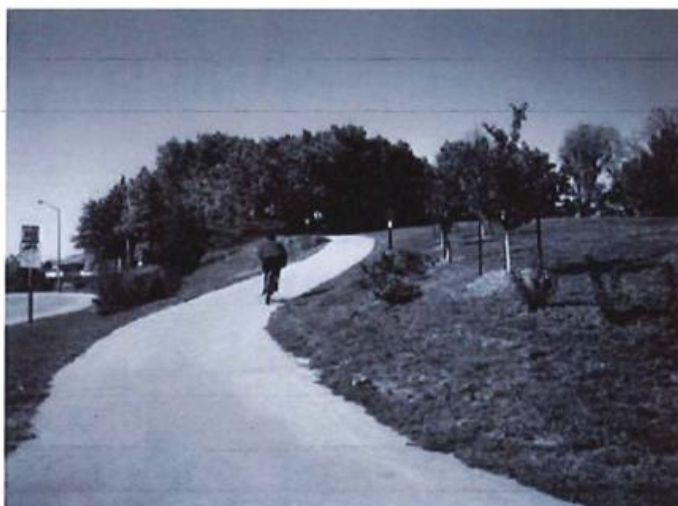
Figure 4-27: Shared-use paths should be designed for all ages. Grades should be carefully considered and should be safe for kids riding coaster brake bicycles.
