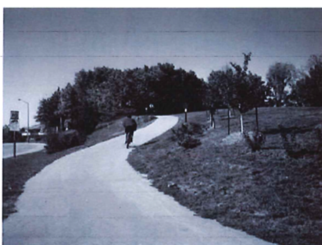
Figure 4-27: Shared-use paths should be designed for all ages. Grades should be carefully considered and should be safe for kids riding coaster brake bicycles.
