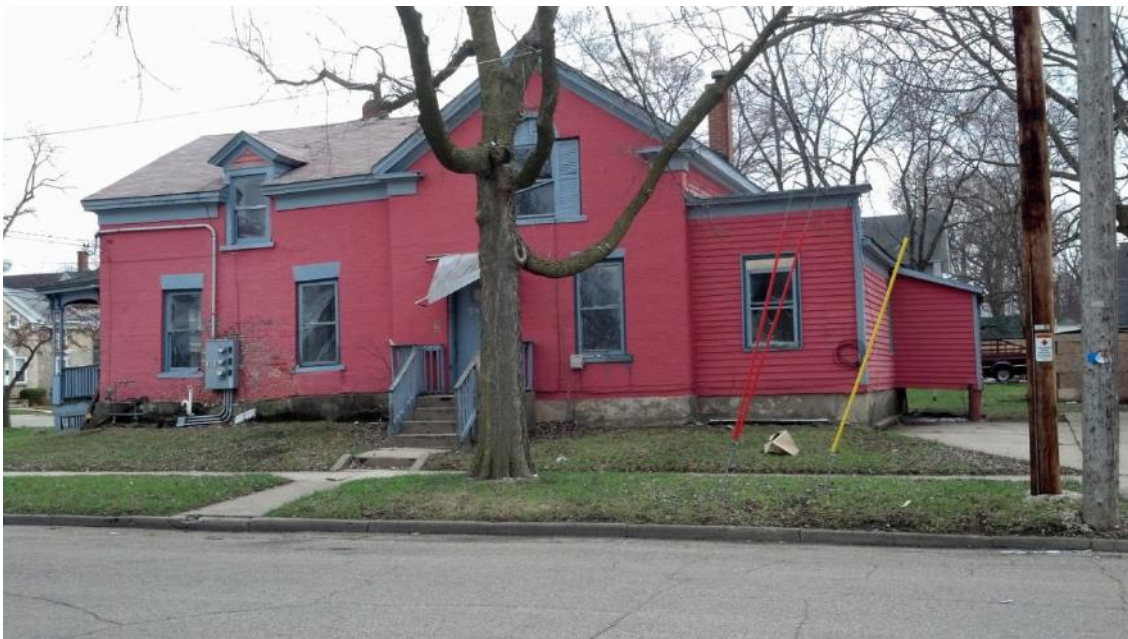
422 Bluff Street - North Side
