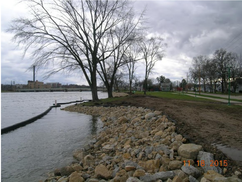
Westside of the Rock River North of the Portland Avenue Bridge
