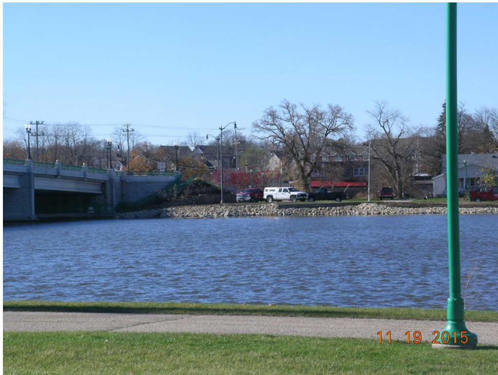
Photo Taken from the East Side of the Rock River Rip Rap along Second Street North of the Portland Avenue Bridge
