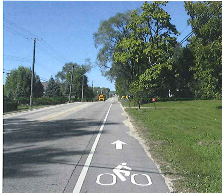
Existing on-road segment in the Town of Beloit.
