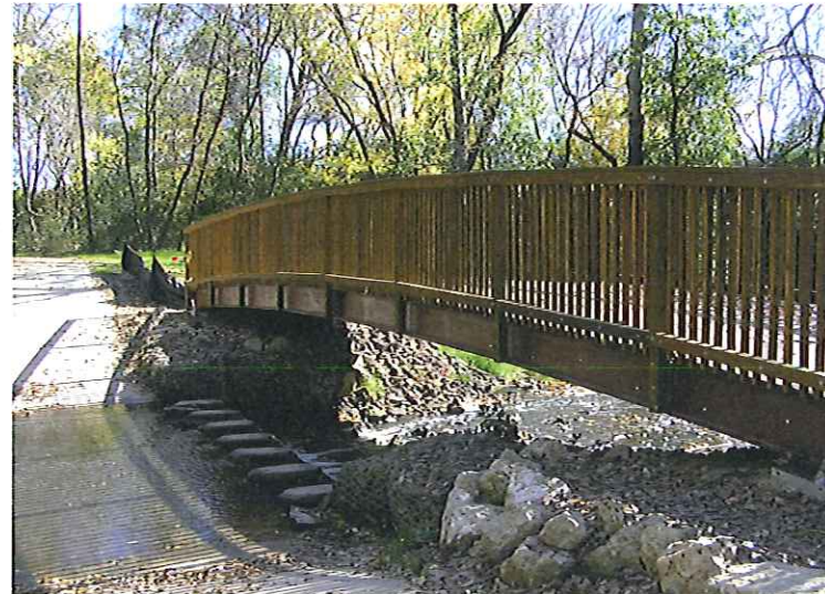
Image of prefabricated bridges that can provide ADA compliant access within trail system.
