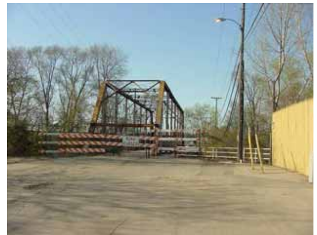
The Wheeler Bridge is a recommended bicycle and pedestrian crossing.
