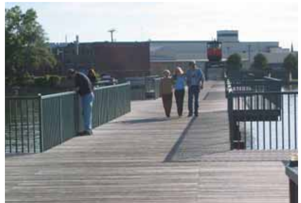
This bridge provides a separated crossing of the Rock River for pedestrians and bikes near downtown Beloit.
