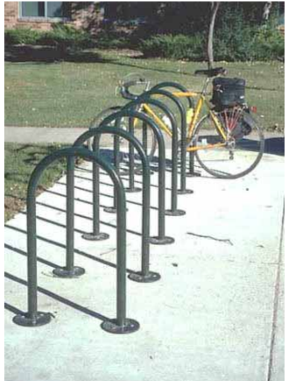
Figure 1: The standard U type bike rack supports the bike frame at two locations and allows users to secure their bikes with either a cable or a U type lock.
