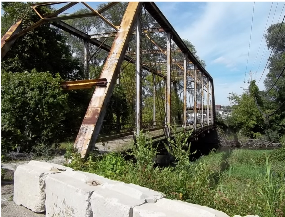
Wheeler Avenue Bridge over Turtle Creek in South Beloit
