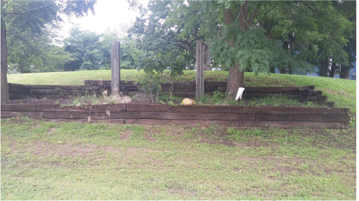
Photo of Existing Sign Posts Intersection of Shirland Avenue and Bluff Street
