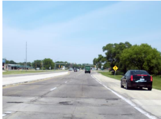
IL-251 Pavement Conditions
