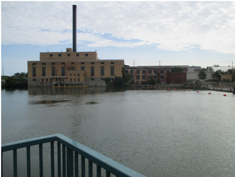
Powerhouse Riverwalk Project, Construction 2018
