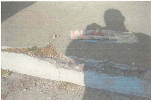
Above left can be seen the damaged concrete on the front steps, revealing a portion of the underlying paver bricks. Above right is a view of the internal section of the porch.
