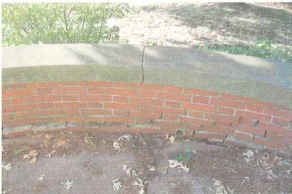
Above left is another view of the inside curve of the front porch. Above right the color of the mortar can be seen to be darker in the protected areas, having been originally colored with coal dust.
