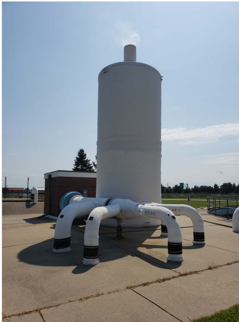
Figure 3.03-4 Mist Scrubber Odor Control System
