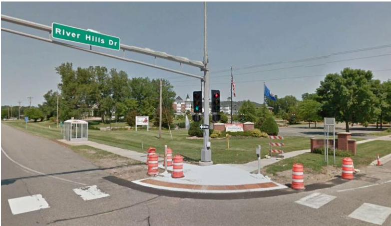
Figure 29. Figure 1: Retrofitted Bus Stop (Burnsville, MN)
