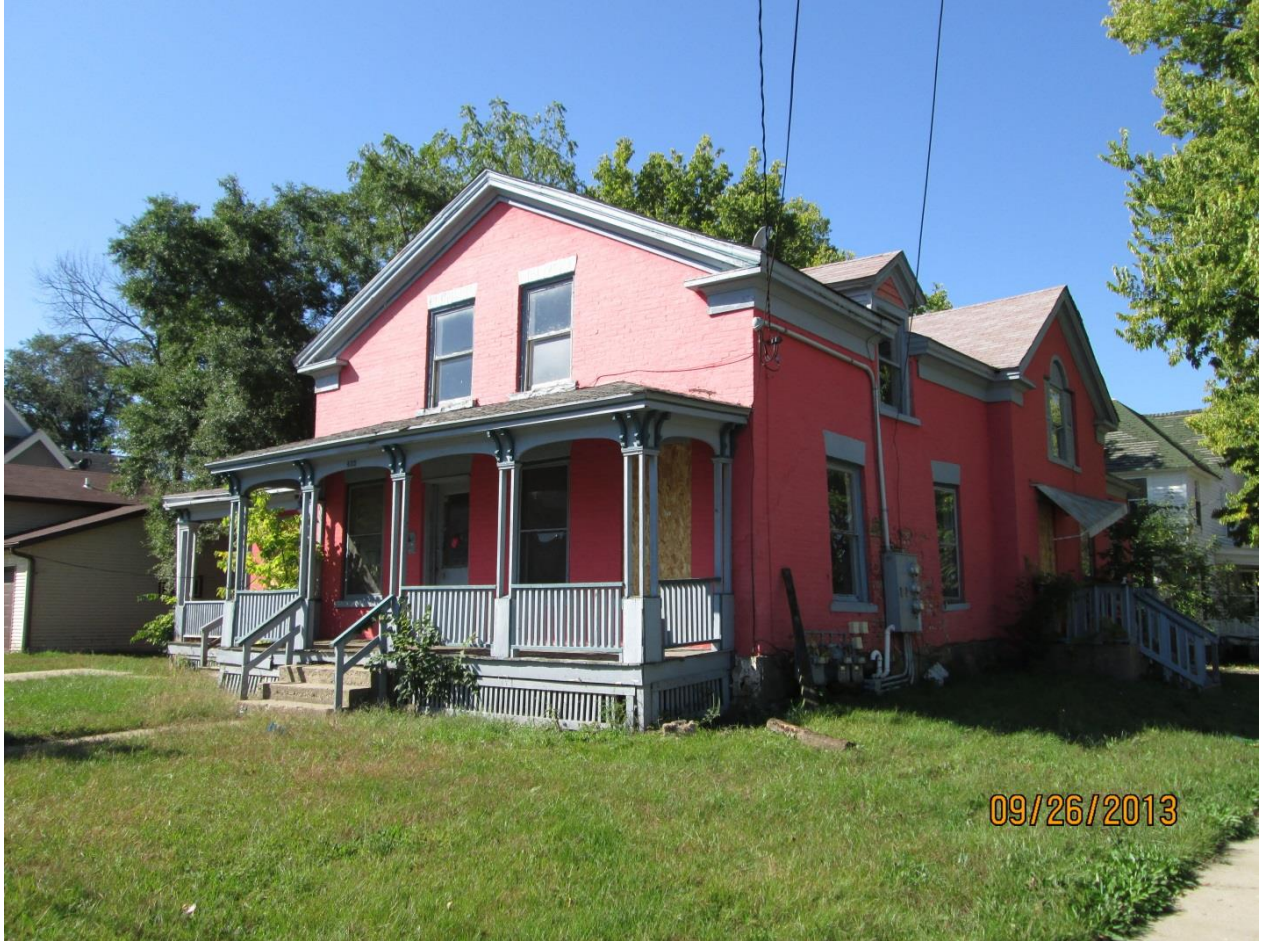
422 Bluff Street – East Side
