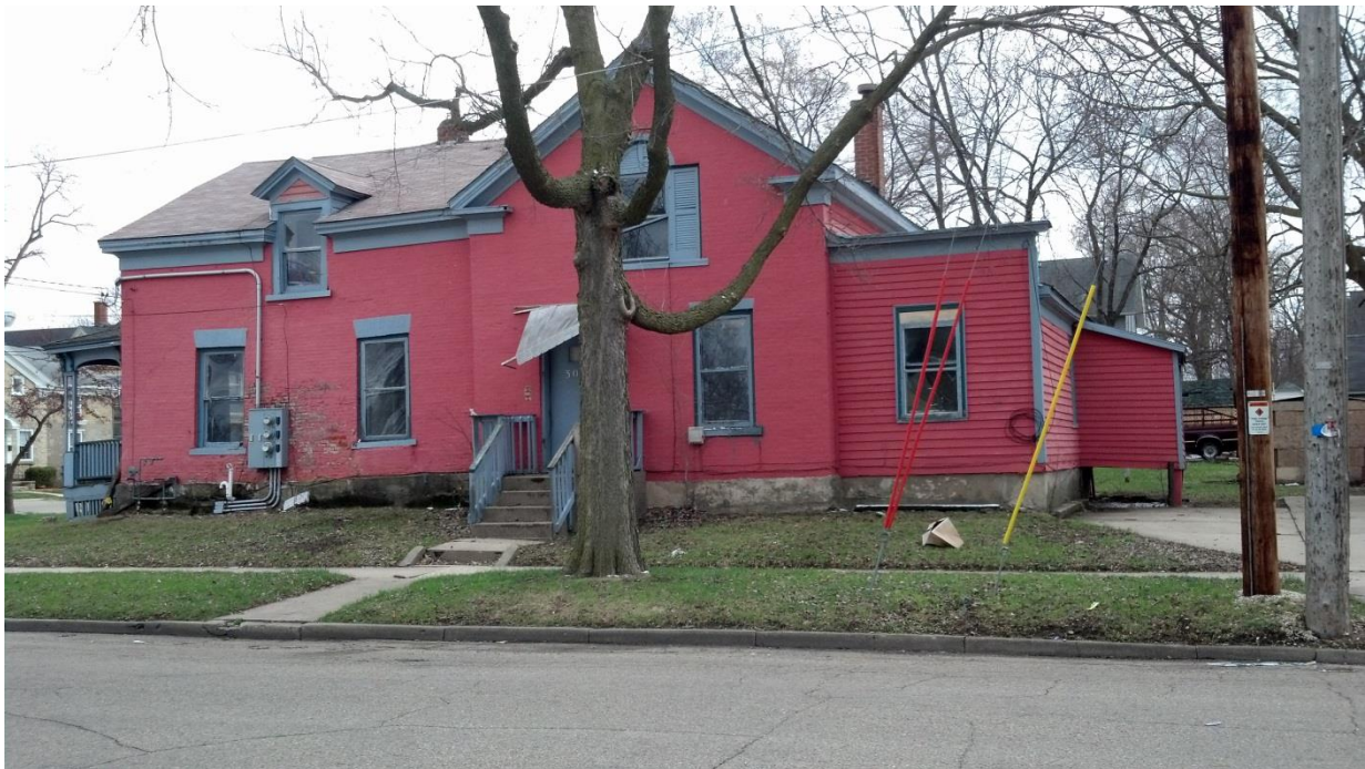
422 Bluff Street – North Side
