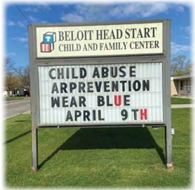
Remove header cabinet and reader board and scrap
