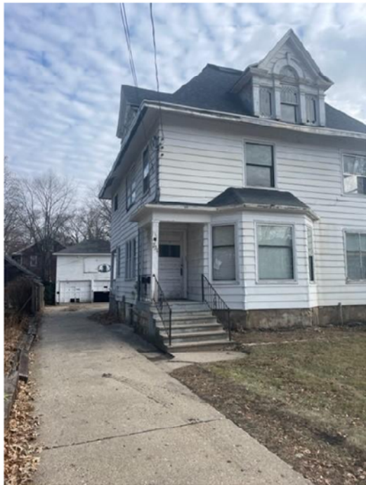
721 Park prior to aluminum siding removal
