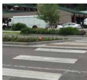
Median refuge island
