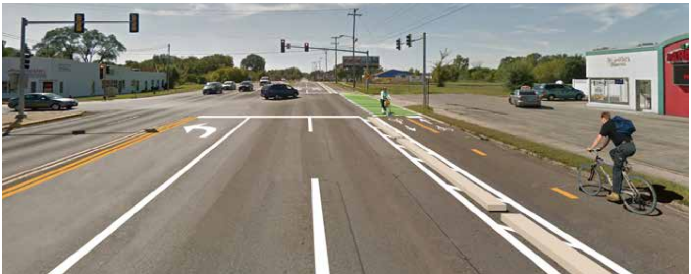
Figure 51. Photosimulation of a two-way separated bike lane on the west side of Blackhawk Boulevard.
