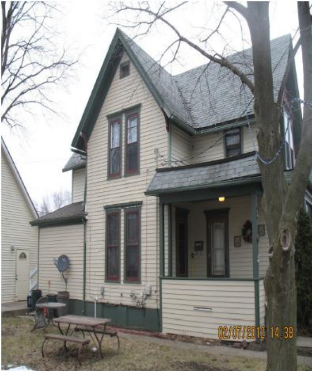
Southern side of house where upper and lower windows will be replaced with proposed new windows.
