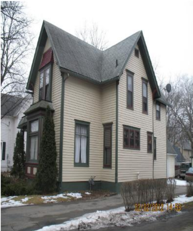
Northeast side of house where one window will be replaced.
