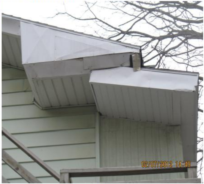
Soffit and fascia panels on the northeast side of the property.
