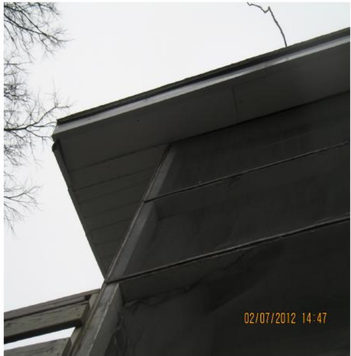
Soffit and fascia panels on the northeast side of the property.
