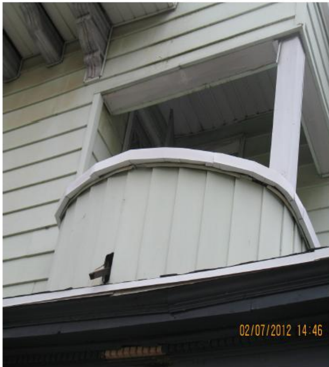
Replaced trim on balcony on the northeast side of the property.
