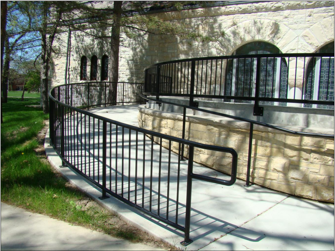
Handrails of Eaton Chapel
