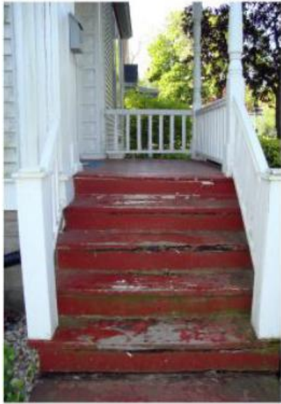
FRONT PORCH (LEFT: Step entry from driveway; RIGHT: detail of spindles)
