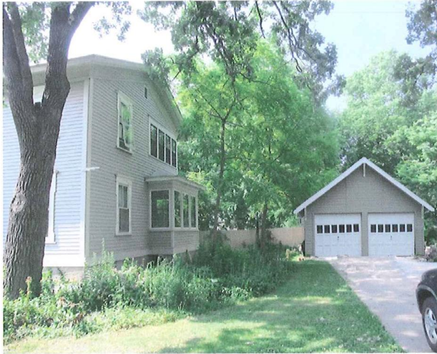
Approximate appearance of the finished garage. Doors will be natural wood, and there will be a small window in the gable.
