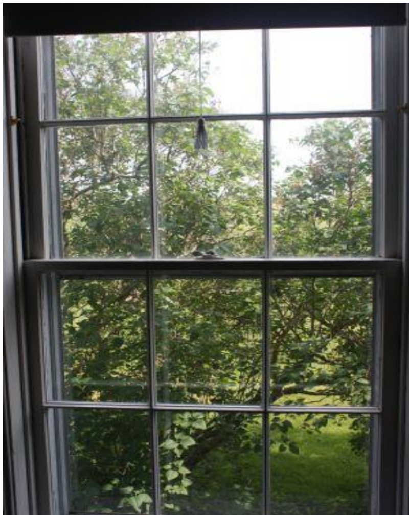
Example of Double-hung Window Applicant is Looking to Secure
