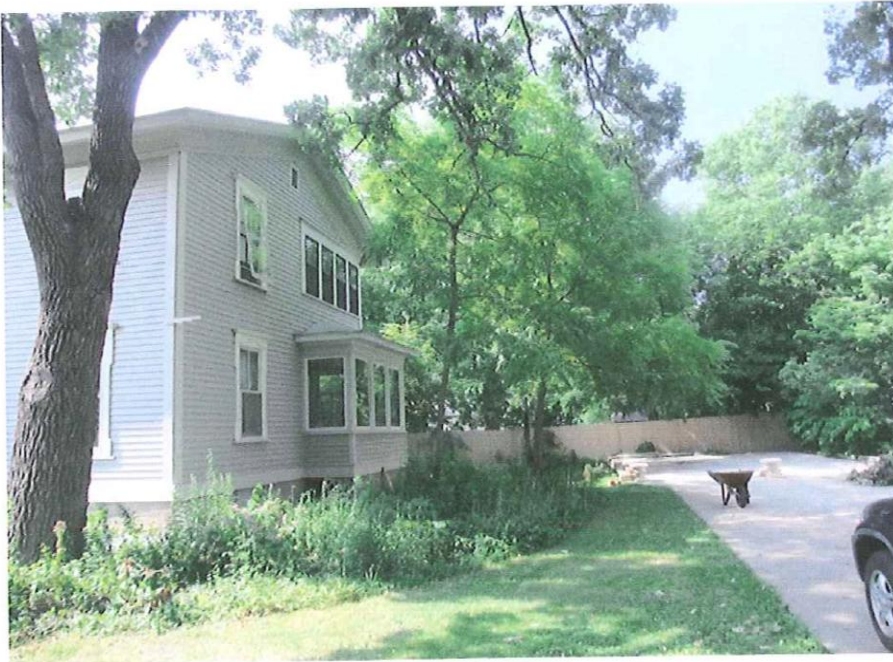
Current Garage slab and siting.
