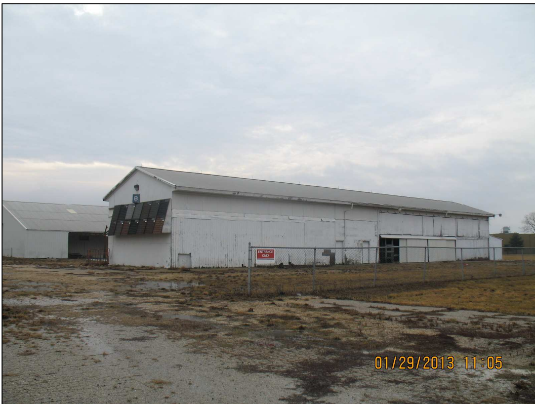
Detached Accessory Structure a/k/a Building “B”
