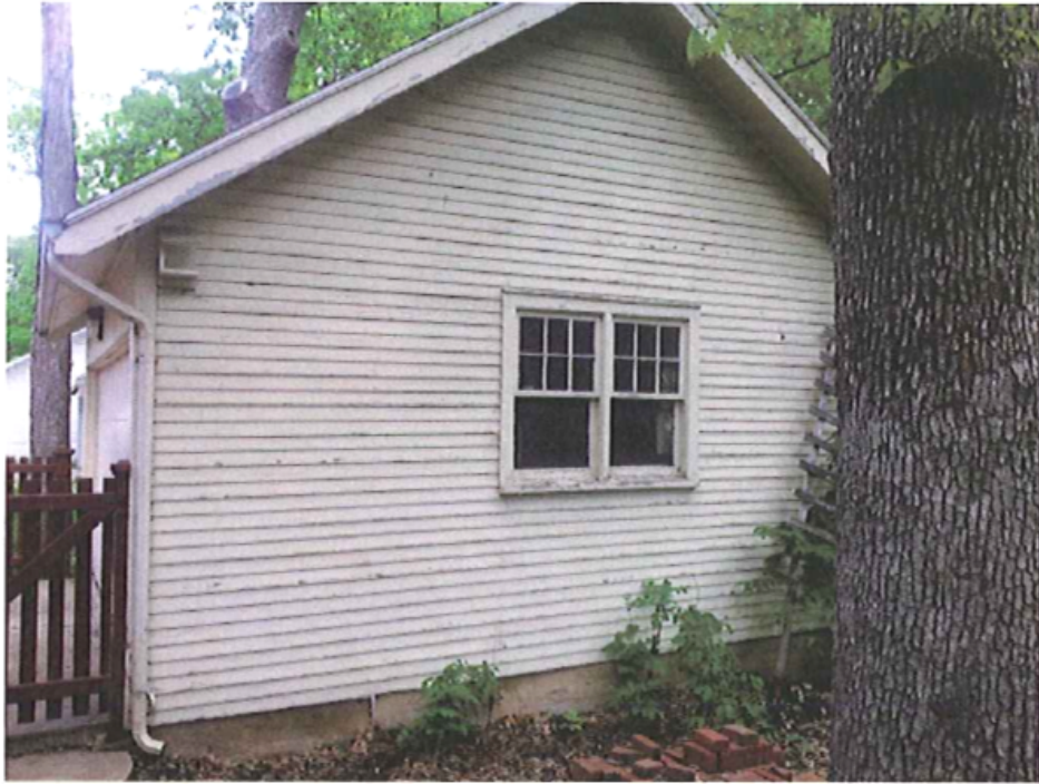
existing garage, south side
