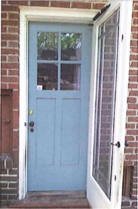
existing exterior house back door
