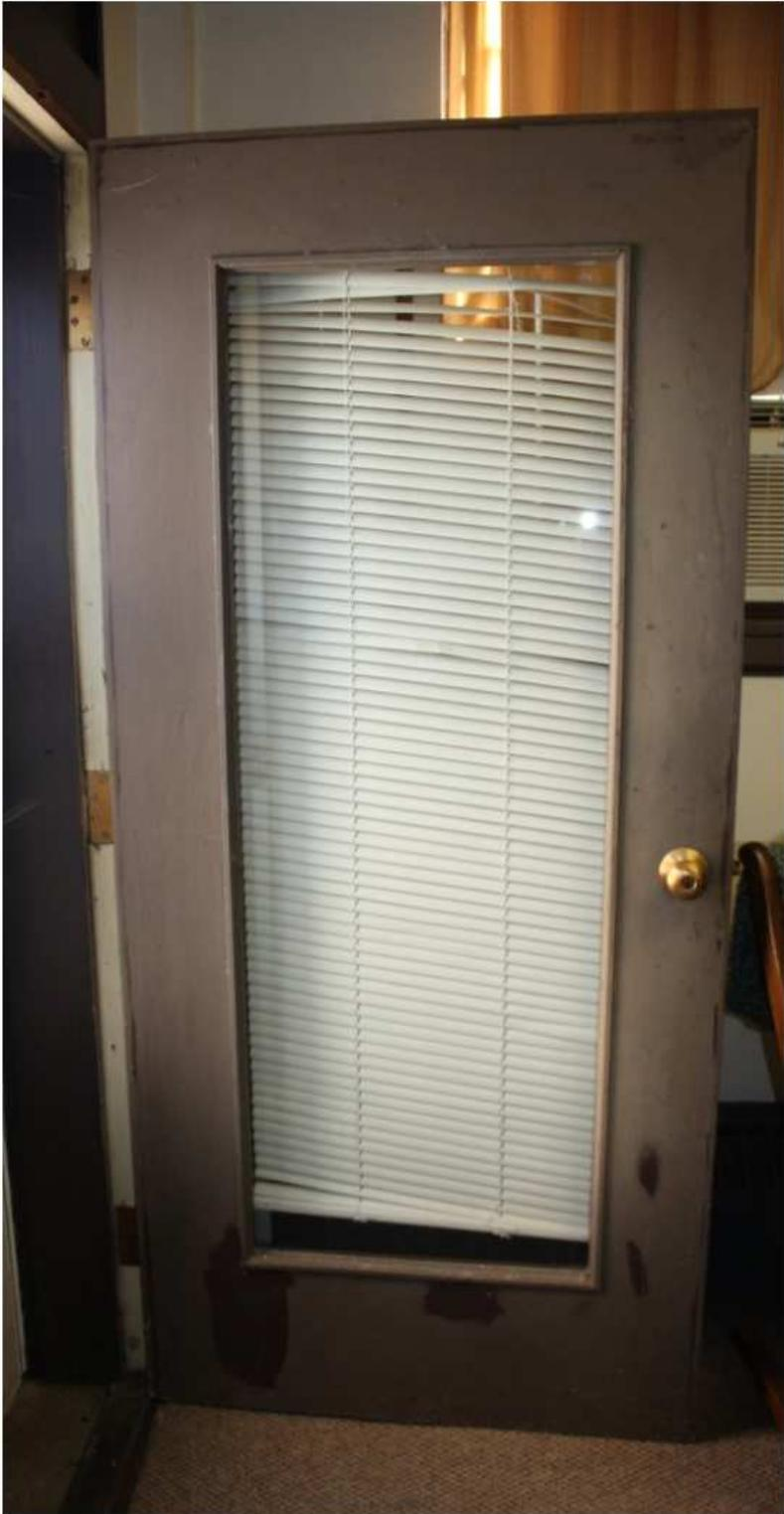
Door in Rector's office that will have glass panel replaced with thermopane panel.
