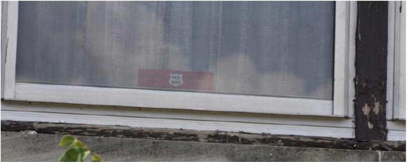
East side 1st floor window showing dry rot
