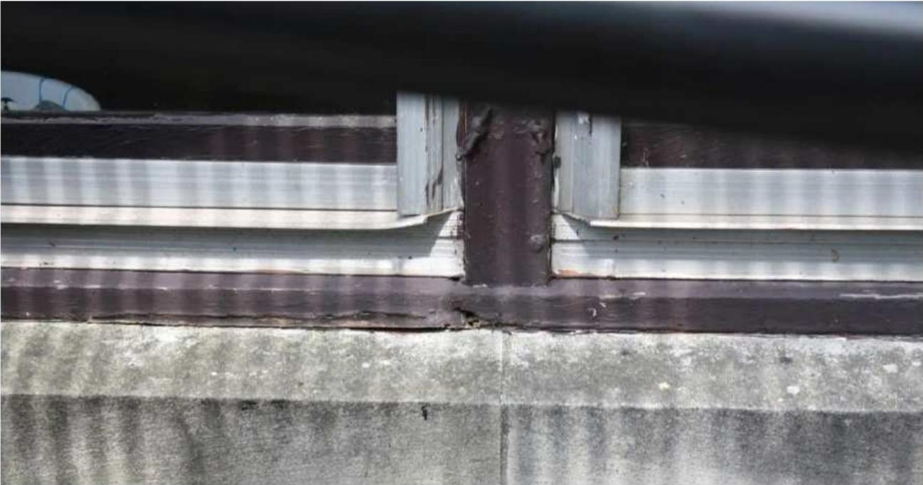
South side 1st floor behind fire escape, sill damage
