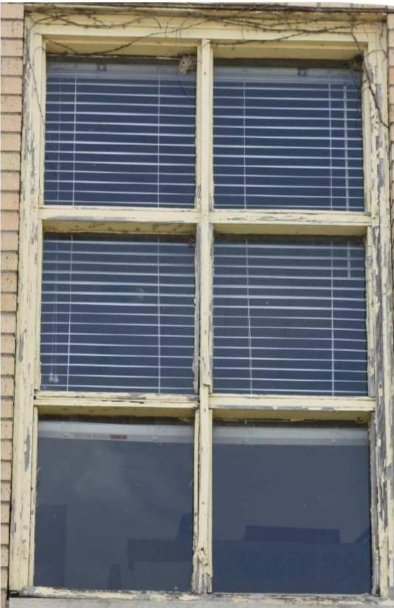
East side landing window showing dry rot and wood damage
