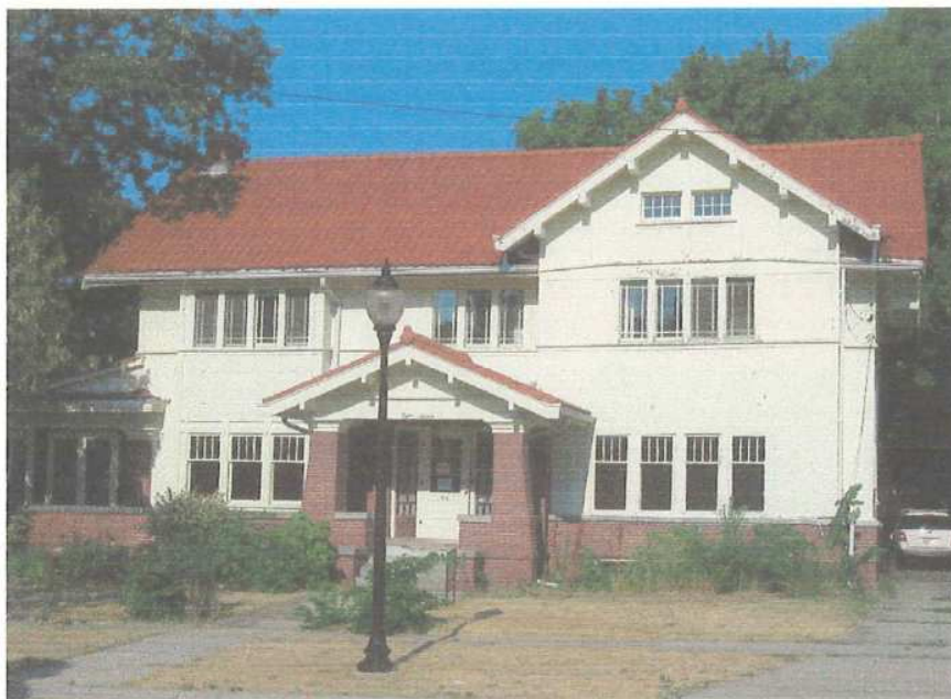
Front (east) view of residence
