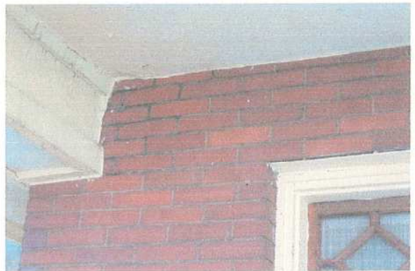
Above left is another view of the inside curve of the front porch. Above right the color of the mortar can be seen to be darker in the protected areas, having been originally colored with coal dust.
