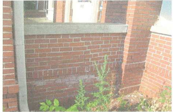
Above left shows the portion of the front porch that was previously deconstructed and improperly reconstructed. The bricks in that section have been painted. Above right is the right side of the porch.
