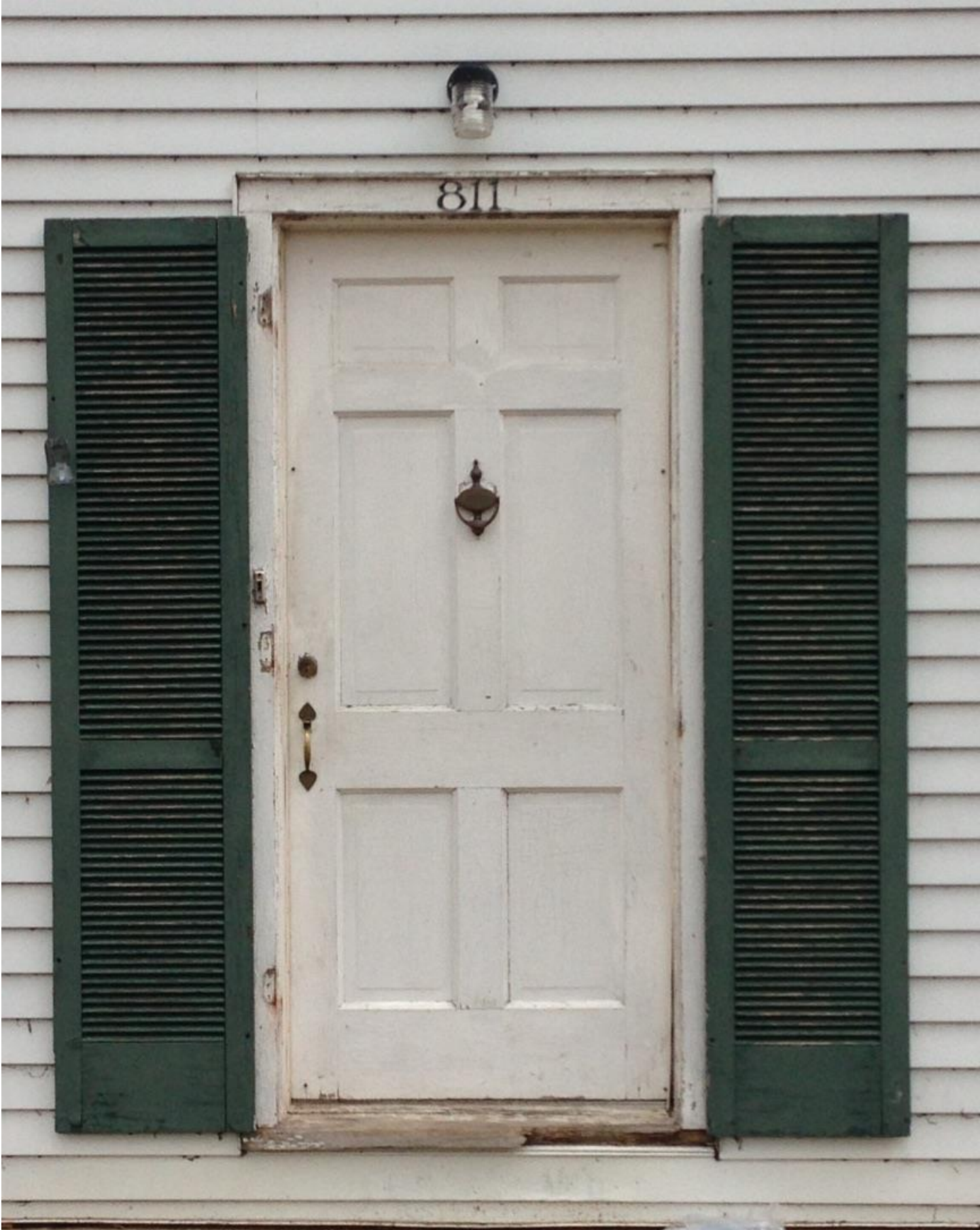
811 Chapin Street – Front Door w/ Shutters
