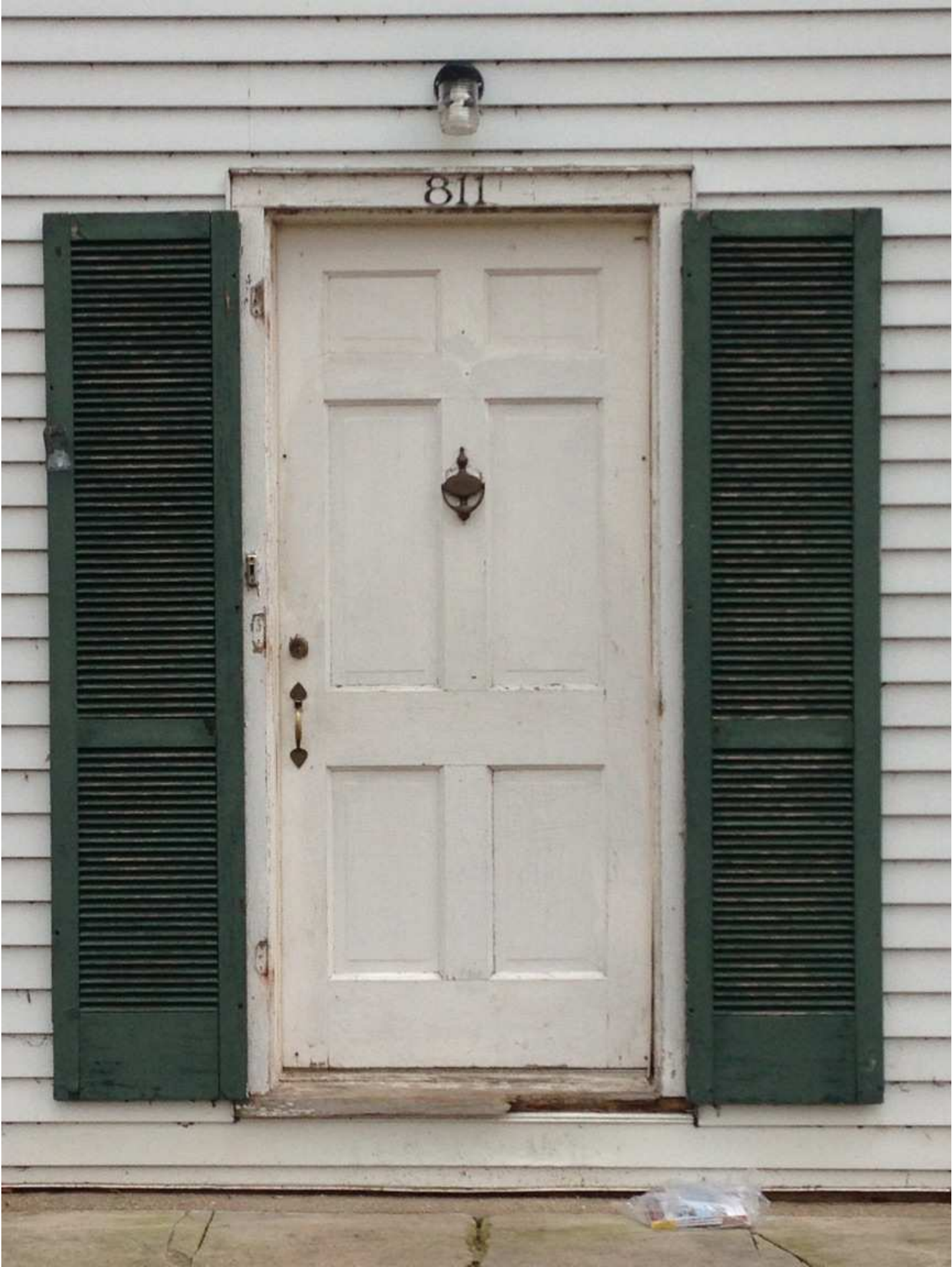
811 Chapin Street – Front Door w/ Shutters
