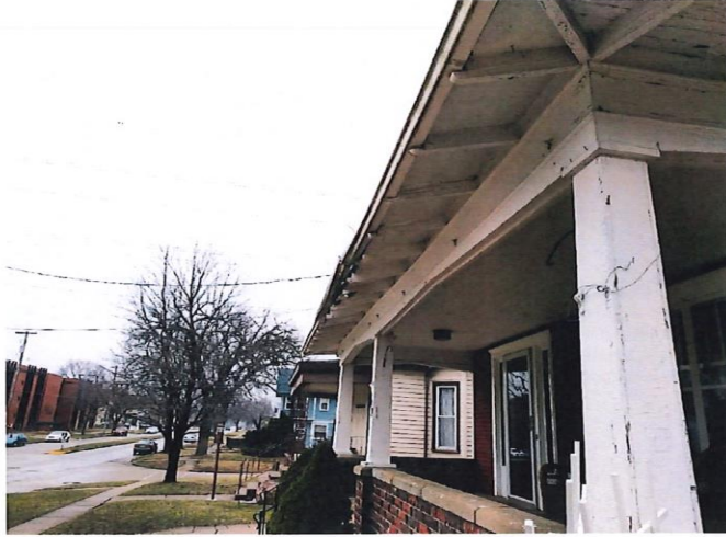
Figure 2: Front Porch Rafter Tails
