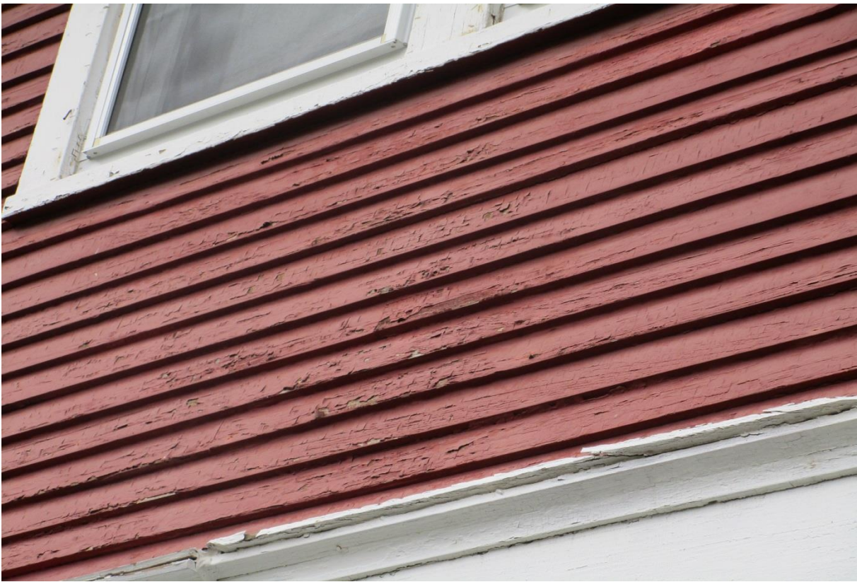
South Side Wall
