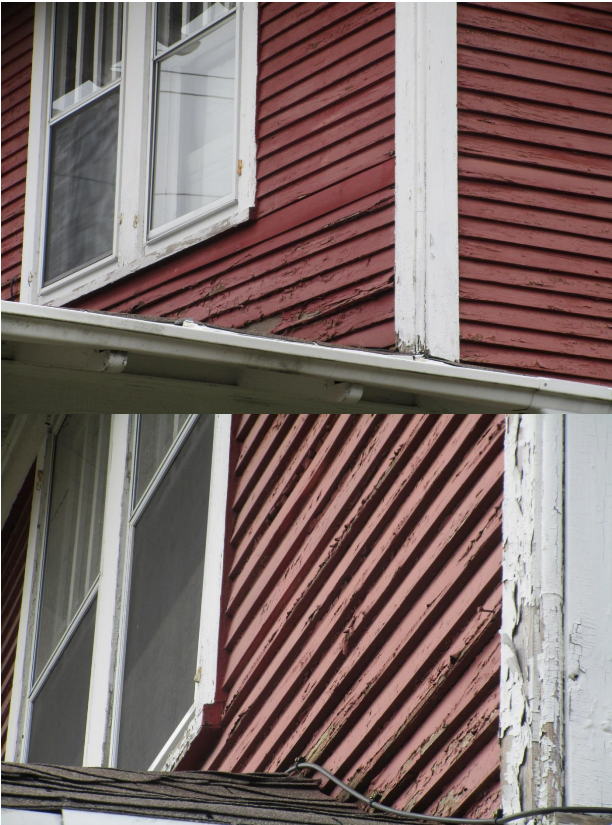
Font Wall (Southwest Corner)
