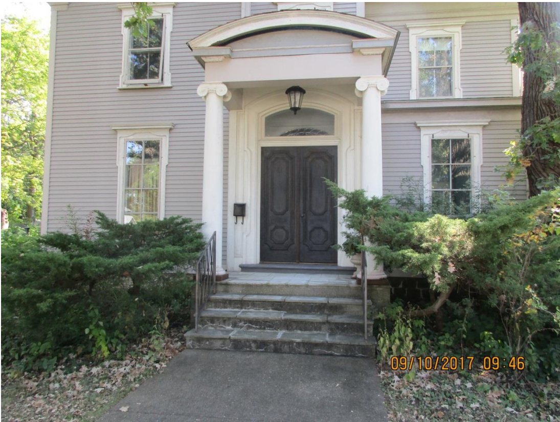
Existing Front Porch
