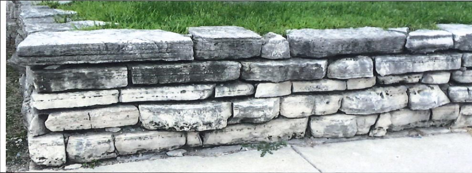
Fig. 4: Example of stacked stone wall.
