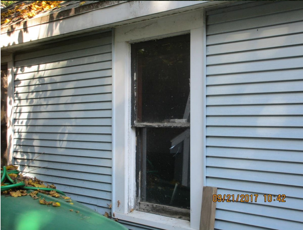
Wood framed windows to be removed.
