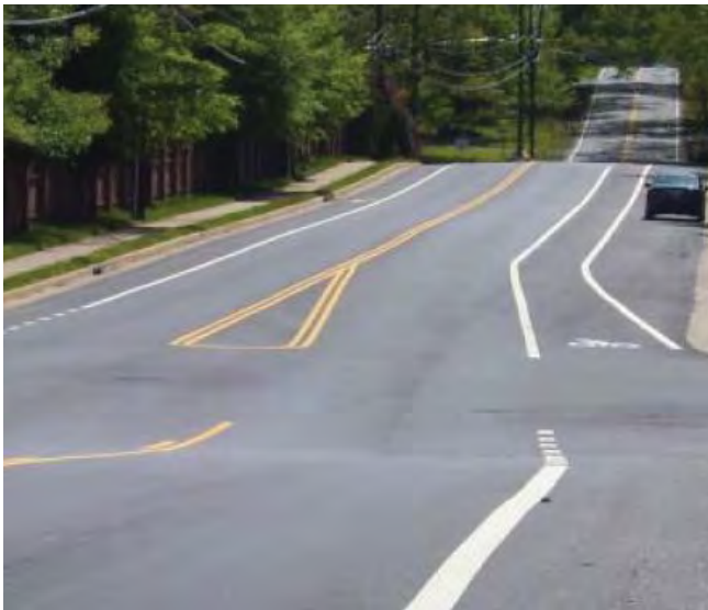
Reconfiguring a roadway to narrow travel lanes and add a center turn lane and bike lanes. Image Credit: Randy Dittberner, Virginia Department of Transportation/FHWA Incorporating On-Road Bicycle Networks into Resurfacing Projects
