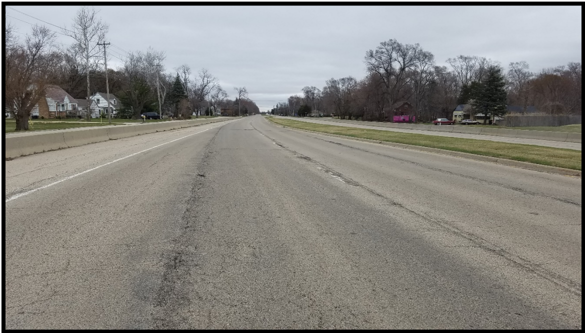
Blackhawk Boulevard southbound lanes, looking north from Prairie Hill Road
