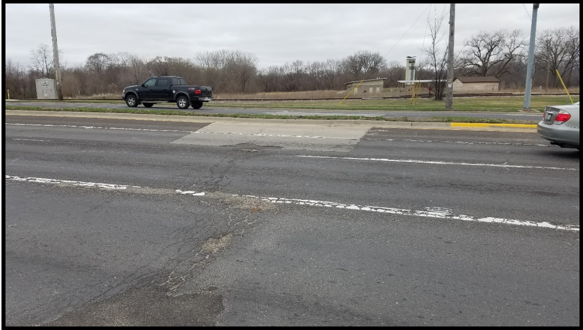
Blackhawk Boulevard northbound lanes at Gardner Street
