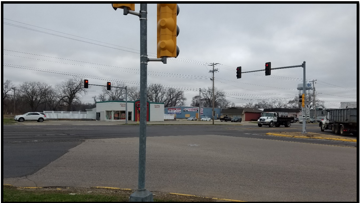
Blackhawk Boulevard and Gardner Street intersection, looking northwest
