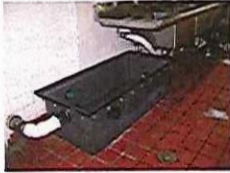
Grease trap after cleaning
