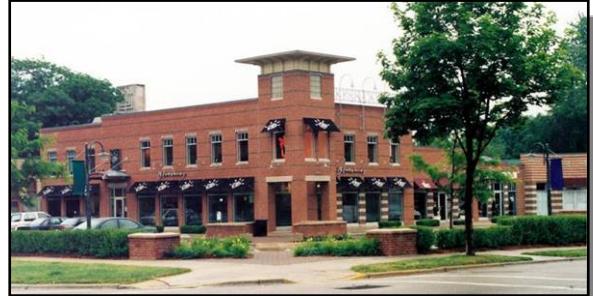
2 nd Highest Score: +1.9 Positive attributes: Building design and placement, parking lot design/ placement
