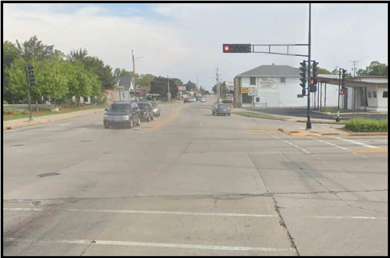
Fourth Street at Portland Avenue, looking south (Source: Google Earth)
