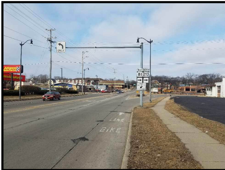
Looking west at Portland Avenue
