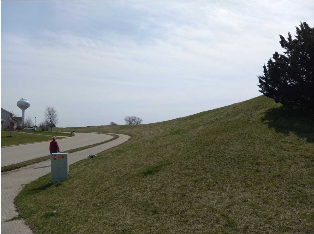
Figure 4: Looking East at Northwest side of site (4/10/2024)
